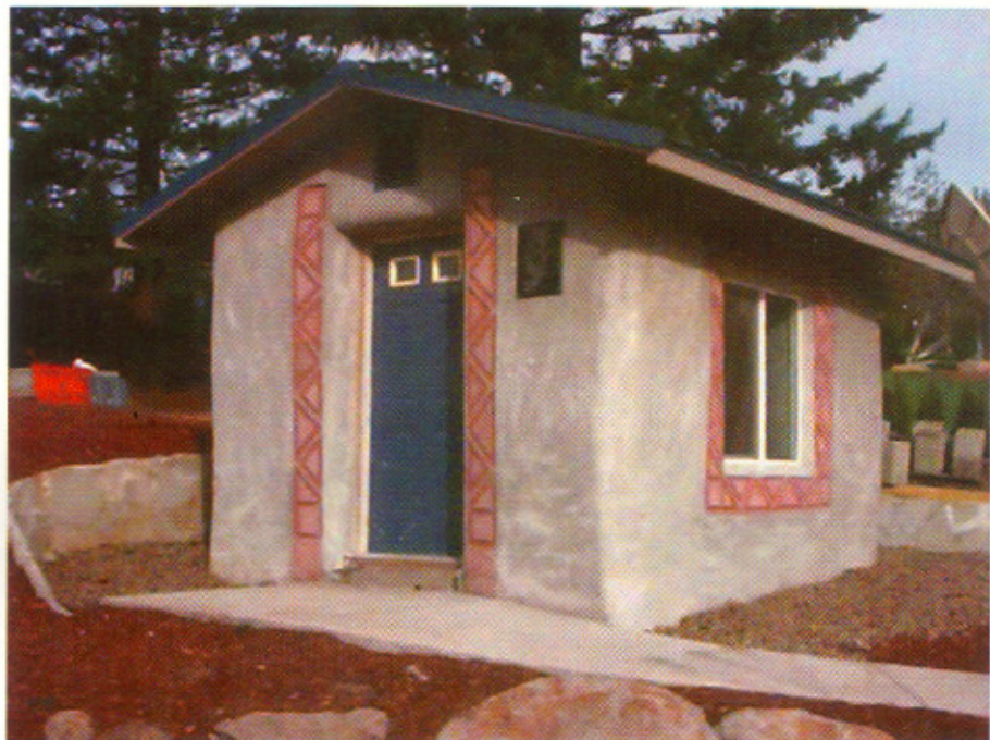
Above: Strawbale test structure at Portland Community College.
